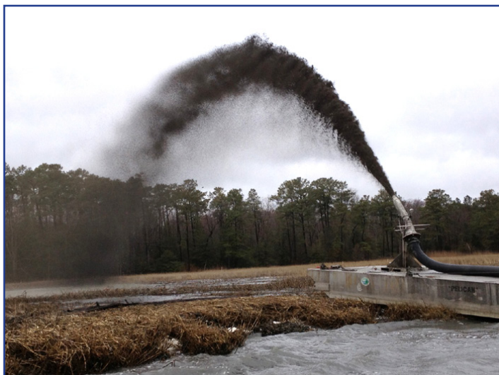
In 2013 the Delaware Department of Natural Resources sprayed dredged sediment on the marshes along Pepper Creek in Dagsboro. The thin-layer spray application promoted the growth of beneficial marsh grasses and will help the marsh keep up with sea-level rise. USF&WS plans to use a similar technique to restore the marshes in the John H. Chafee Wildlife Refuge.
